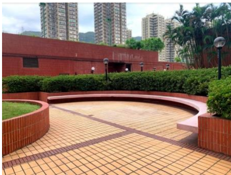
Figure 14. Podium garden at Tuen Mun Town Plaza (Phase I)
