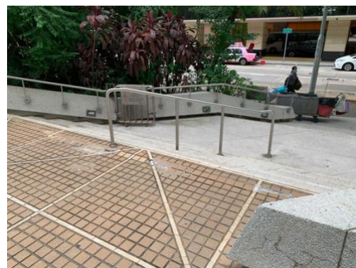
Figure 18. Staircase at the entrance to the POSPD at City Garden
